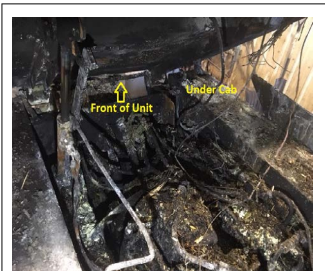
Fire damage under cab
