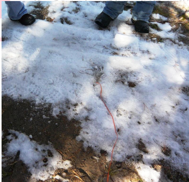
Example of a Loaded Shot Hole with Protruding Wires
