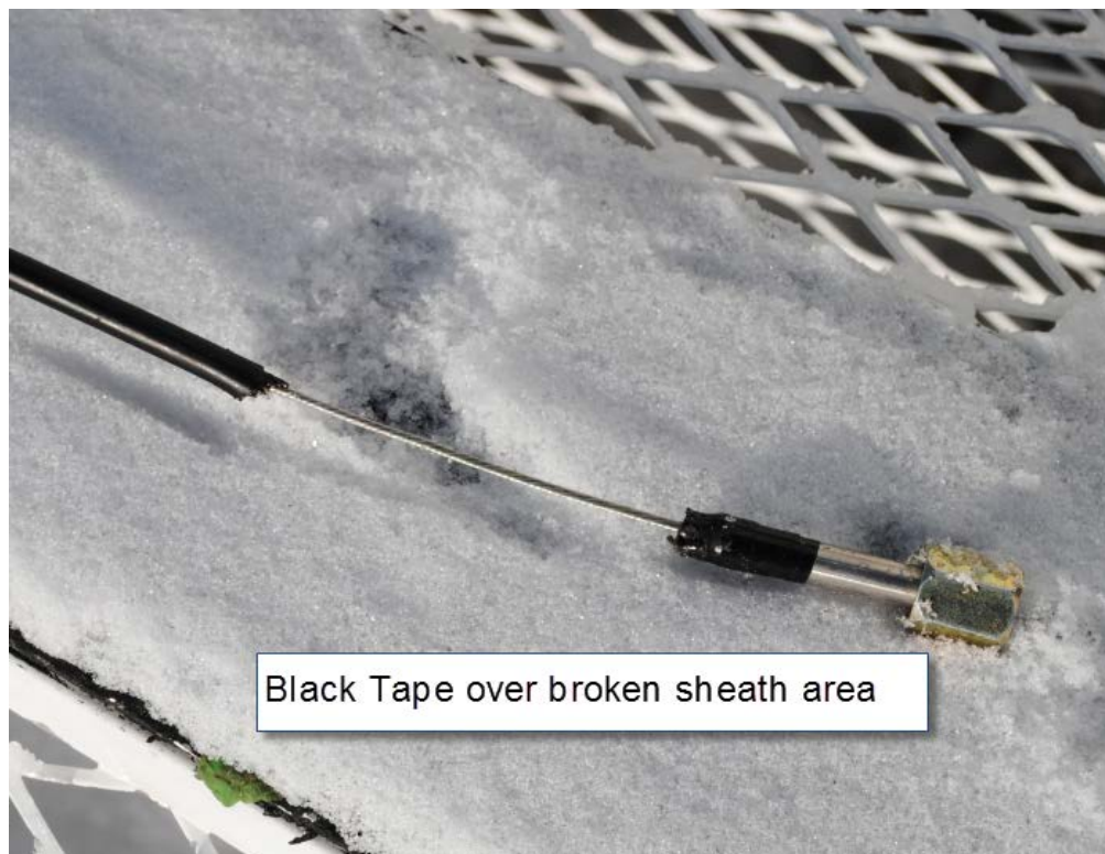
Broken sheath with black tape on
