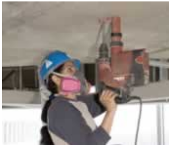
Concrete drill with a HEPA filter attachment.
