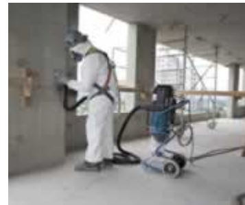
Worker grinding concrete using a HEPA vacuum exhaust attachment on the grinder.
